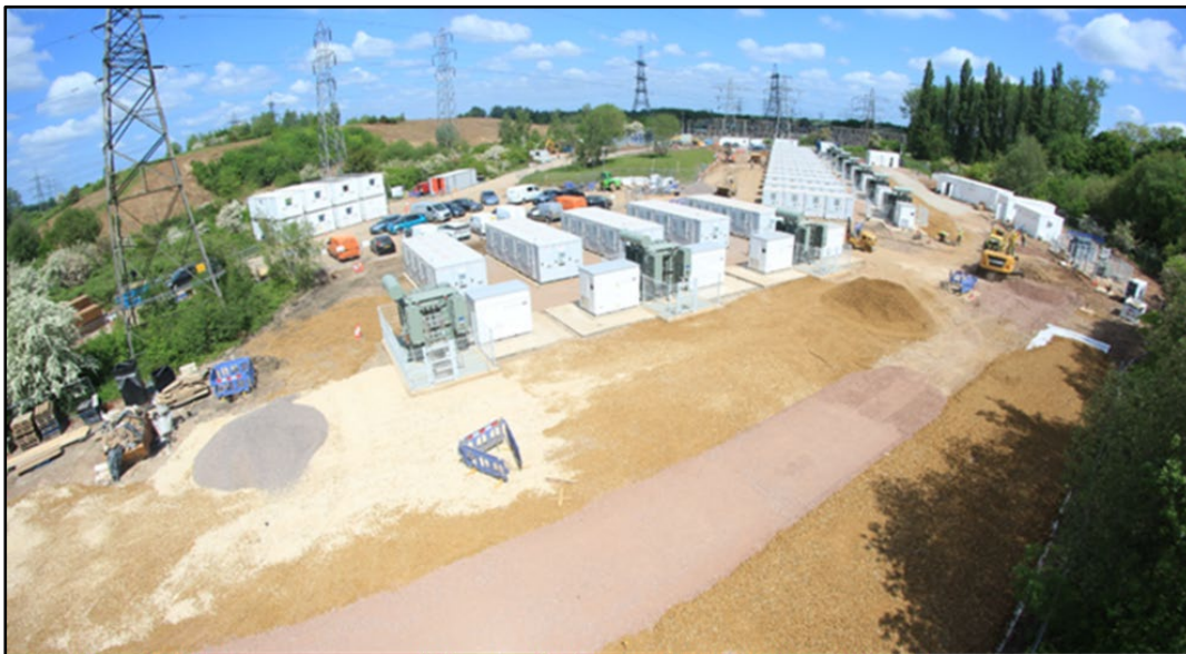
Plate 3.10: Example of the construction of BESS Compound
