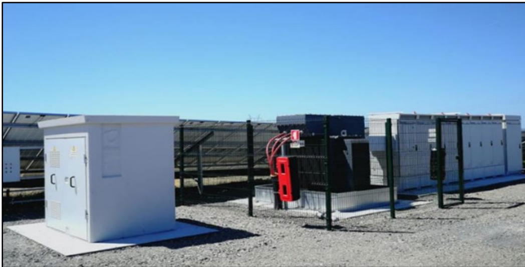
Plate 3.4 Typical Independent Outdoor Equipment (left to right: Switchgear, Transformer, Central Inverter)
