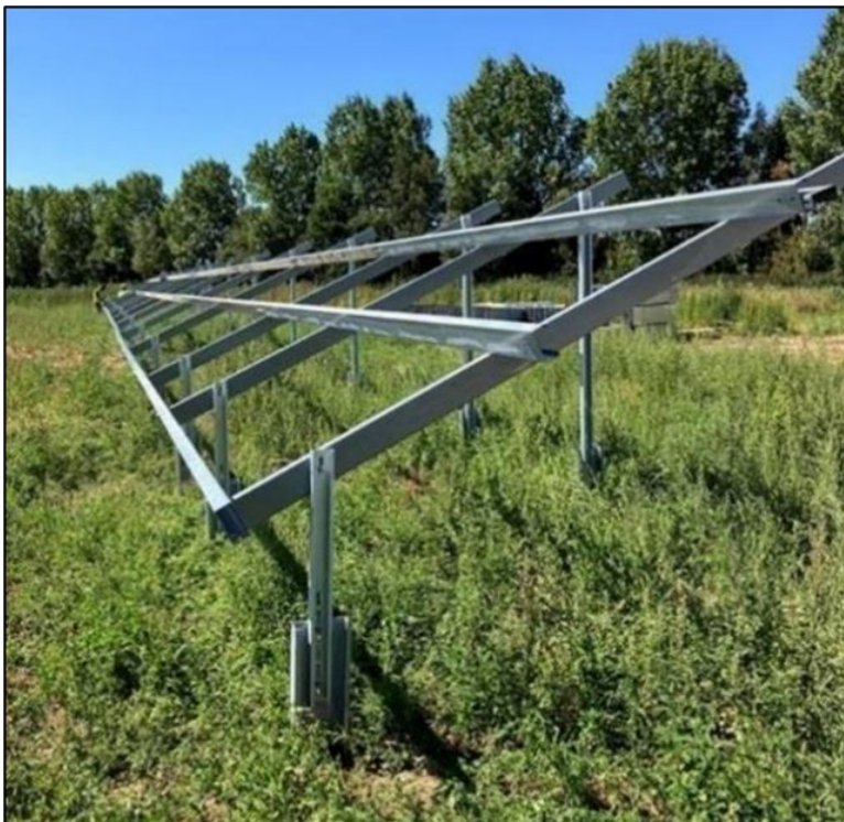
Plate 3.13: Example Solar PV mounting structure
