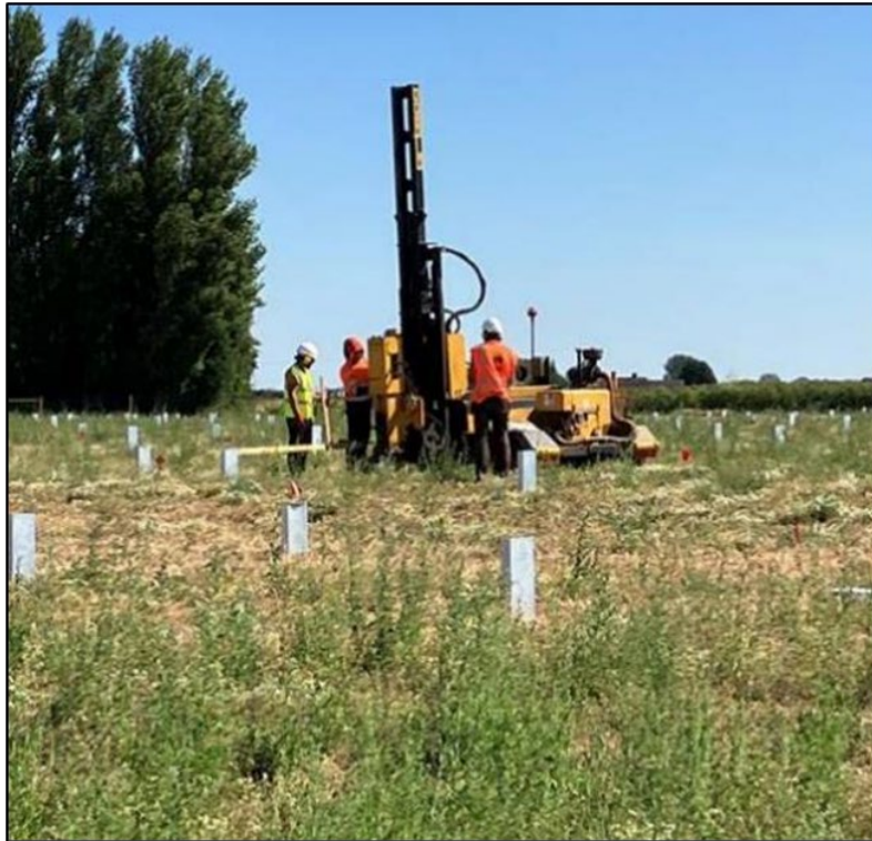
Plate 3.14: Example construction piling for the installation of the Solar PV mounting structures
